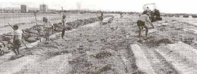
Hand spreading of mulch on Wave Break Island (Source: GCCC 1986)
